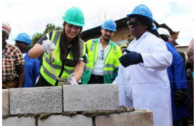
Women build in Bauleni
